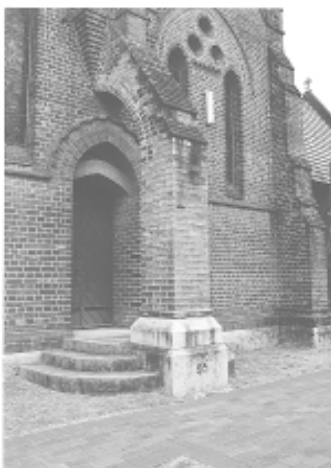
Flying buttress on the northern side
