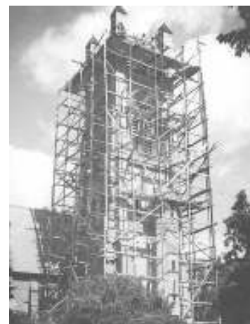
Tower under construction
